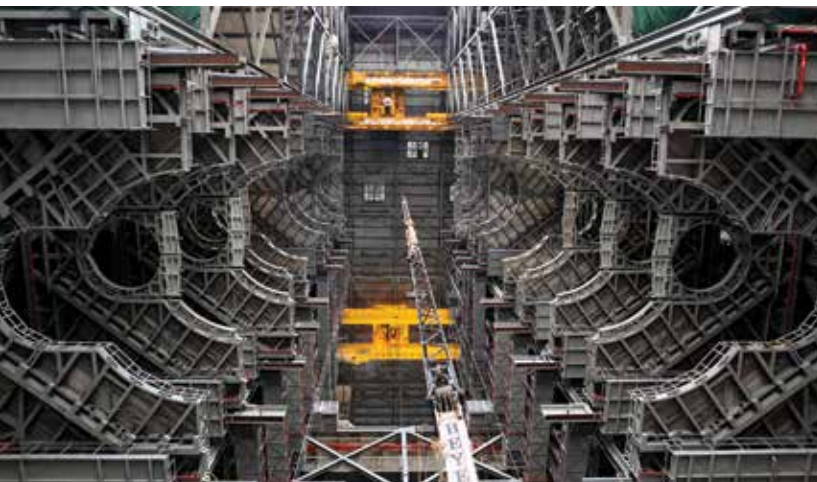
Final work platform installed in Vehicle Assembly Building for Space Launch System. (NASA/Frank Michaux)
